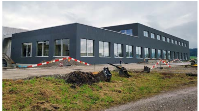
The expansion of the location of Stamm AG in Hallau (CH) was completed.
